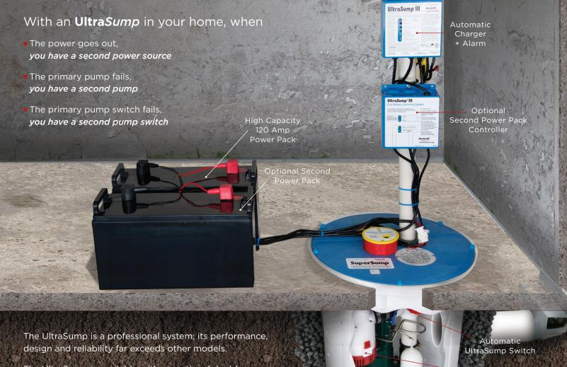
The UltraSump is available with an optional double power pack configuration (shown) to double the total gallons it can pump out. Ask your dealer for more information.
