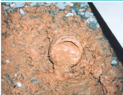
DRAIN PIPES CLOGGED WITH IRON OCHRE
