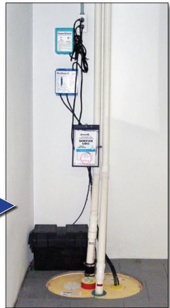
*If the power to the circuit is lost, the PowerWatch<sup>™</sup> will inform the homeowner either, through an audible alarm, or remotely through your home security system input, that power has been lost to that circuit. (Security system tie-in not included.)*
