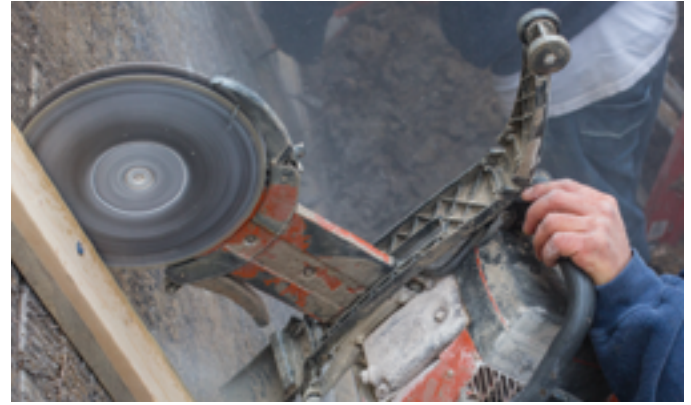
Above | The cut-n-break saw is designed specifically for making clean, accurate cuts through foundation walls.
