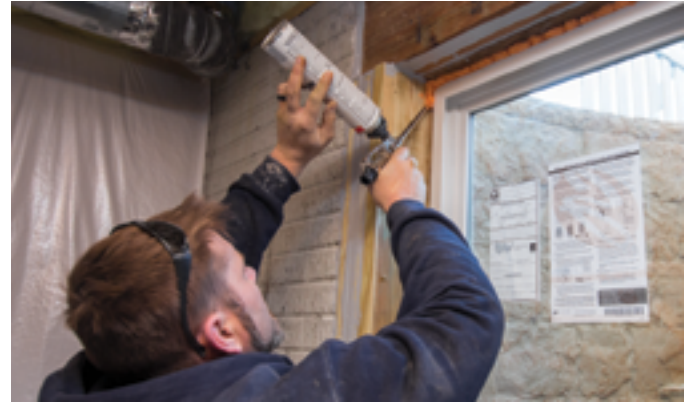
Above | A properly sealed window keeps the elements out and conditioned air in.
