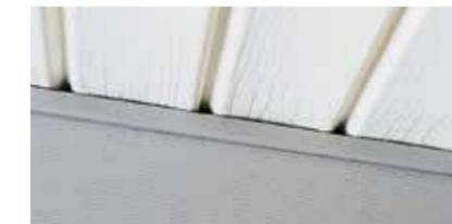
*Ordinary soffit lacks stiffness, so it tends to cup when installed.*
