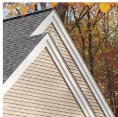
*5" Trimworks lineals used as "rake" boards.*
