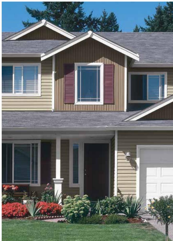
*Unvented Charter Oak soffit panels used as vertical siding, create a focal point above the main entrance. The vertical lines also interrupt long horizontal lines that could tend to make the home look "stretched out".*
