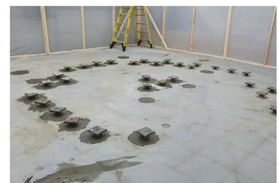
Completed Helicast piles to be embedded within the concrete foundation
