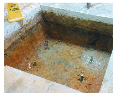
One of six pile cap excavations with HA175 helical piles installed
