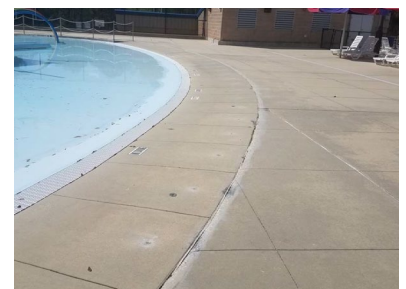
Pool edge slabs after PolyLevel injection
