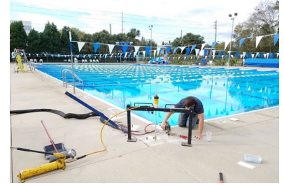
Installing PolyLevel around pool edges with lift assist tool
