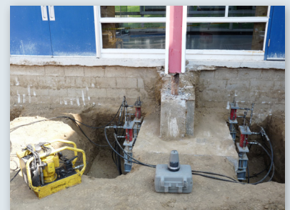
Hydraulic cylinders to apply load to the piers
