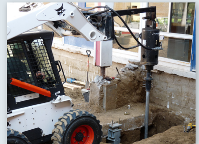
Advancing helical piers adjacent to existing column footings
