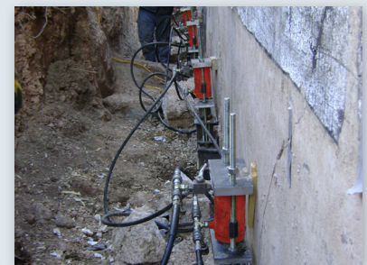
Piers driven to stable soils
