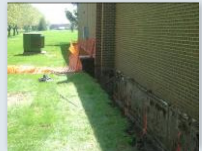
Pier locations marked
