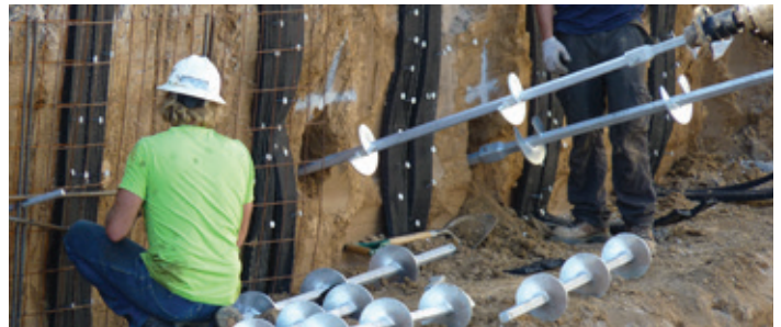
Helical Soil Nail Installation; Placement of Drainage Strips and Reinforcing
