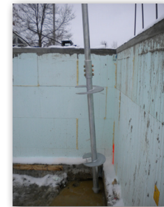
Retrofit pier is advanced
