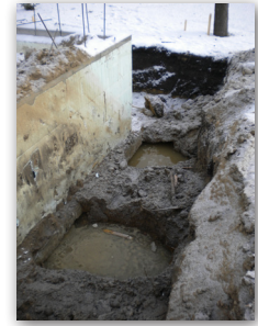
Excavation completed for retrofit pier installation
