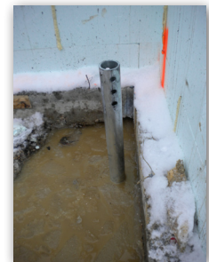
Pier installed and awaiting foundation bracket
