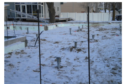
New construction piers installed for concrete floor slab
