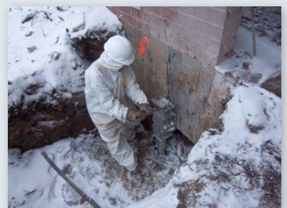
Setting cap plate on the retrofit bracket assembly
