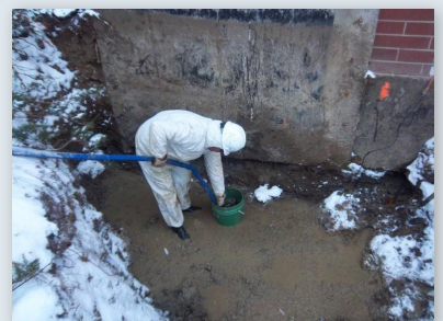
Makeshift sump to keep water levels down
