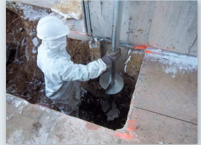
Excavation made for retrofit helical piles
