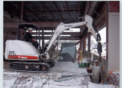
Aligning the drive head with the pile for installation
