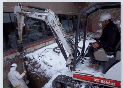
Advancing helical pile
