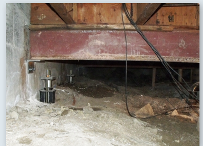
Pier installations completed in tight conditions
