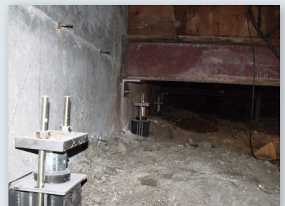
Pier installations completed in tight conditions
