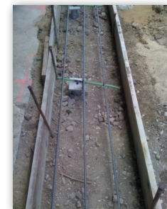
Rebar placed and footing ready for concrete
