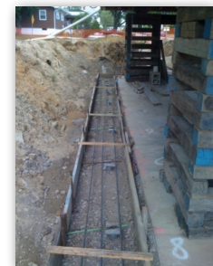
Rebar placed and footing ready for concrete
