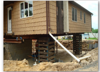
House lifted and original foundation removed
