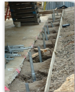
New construction helical piers installed
