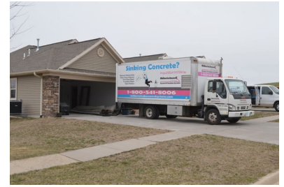
PolyLevel rig at jobsite
