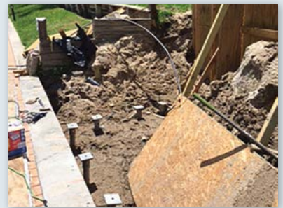
Piles installed and fitted with new construction brackets
