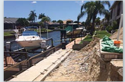
Original retaining wall and pool deck removed
