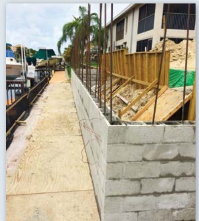
New retaining wall supported by helical piles
