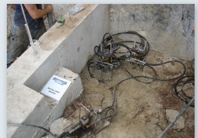
Piers are connected and seating load applied
