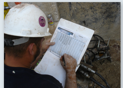
Installation pressure is logged for each pier
