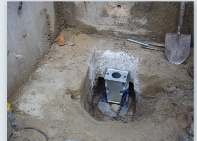
Footing prepared and bracket set
