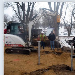
Installation of helical piles
