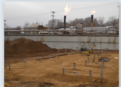
Pile installation complete, placing fill
