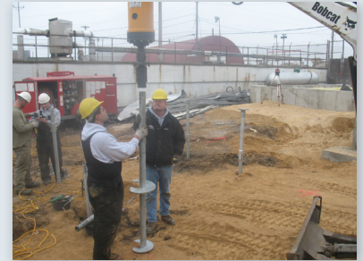
Installation of helical pile lead section
