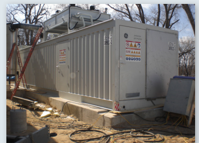
Foundation complete and generator installed
