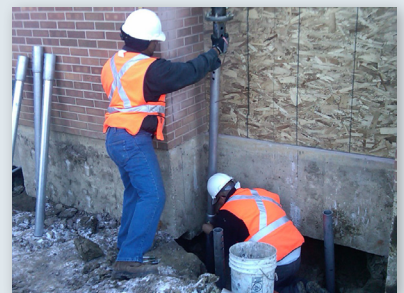
Attaching helical pile extension
