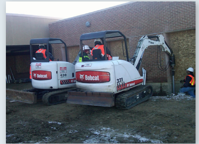
Retrofit helical pile installation
