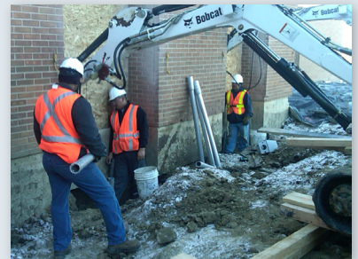
Retrofit helical pile installation
