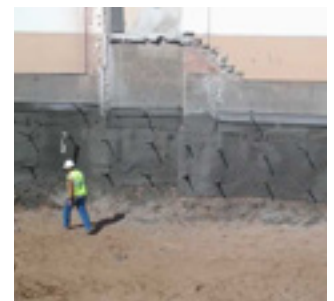
Completed shotcrete wall section
