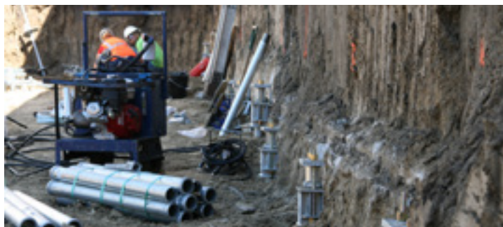
Installed push piers with side-load foundation brackets
