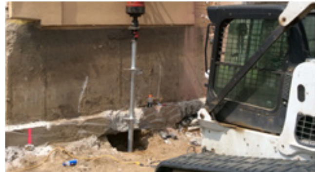
Installation of HP288 helical pile
