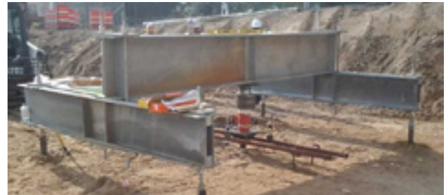
Compression load test on HP288 helical pile
