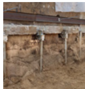
Helical piles and tiebacks after excavation
