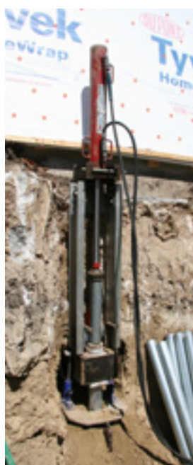
Driving Model 288 push pier
