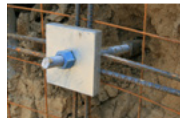
Helical soil nail head detail
