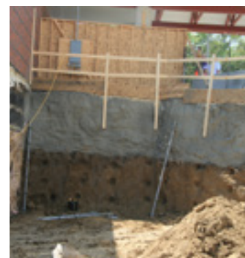
Two-tiered soil nail wall under construction
