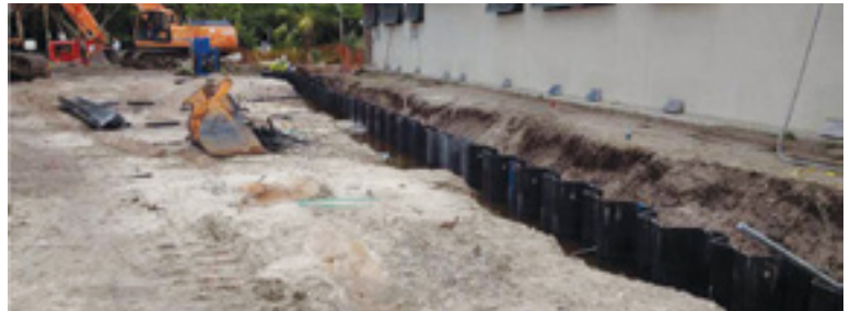
Sheet pile wall installed behind parking garage
