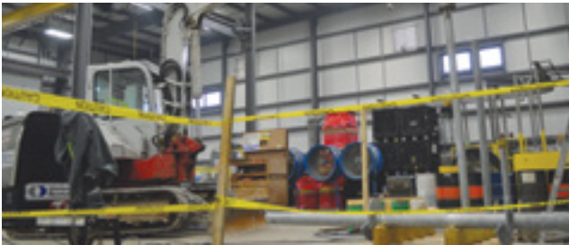
Installing HP450 helical piles with small excavator
