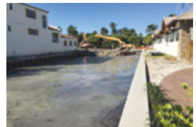
Seawall caps poured and inlet dredged
