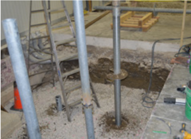
Advancing lead section
