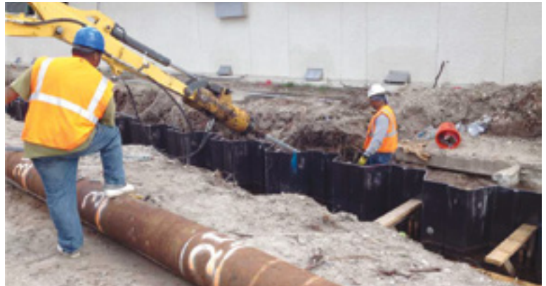
Installing tiebacks from top of sheet pile wall
