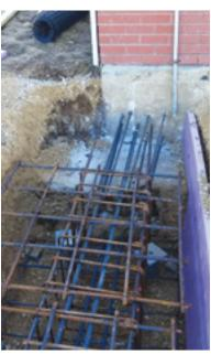
Pile cap and grade beam reinforcement installed around helical piles
