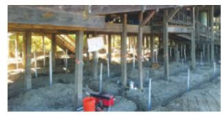
Helical piles installed within grade beams at column locations
