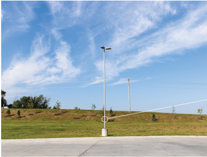
New light pole rusting where inert coating was damaged
