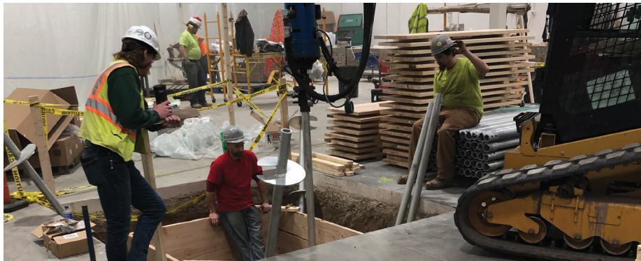
Installing helical piles in pile cap
