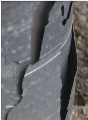
Powder coat flaking off helical pile during low strain conditions of installation
