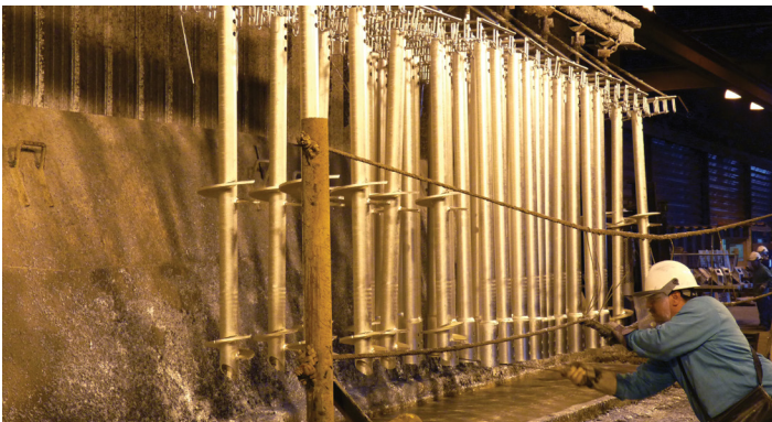
Helical piles removed from the zinc bath
