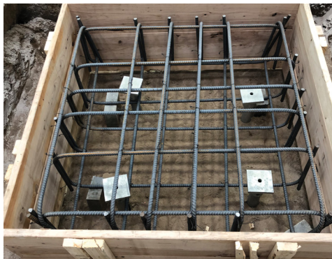
Helical piles with new construction caps and reinforcement
