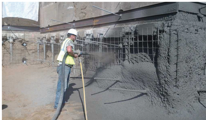
Application of shotcrete facing
