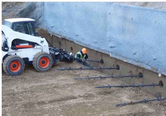
Installation of helical soil nails
