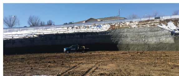
Helical soil nail wall in service prior to building construction
