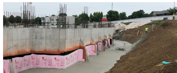
Cellular concrete placed between office building and soil nail wall
