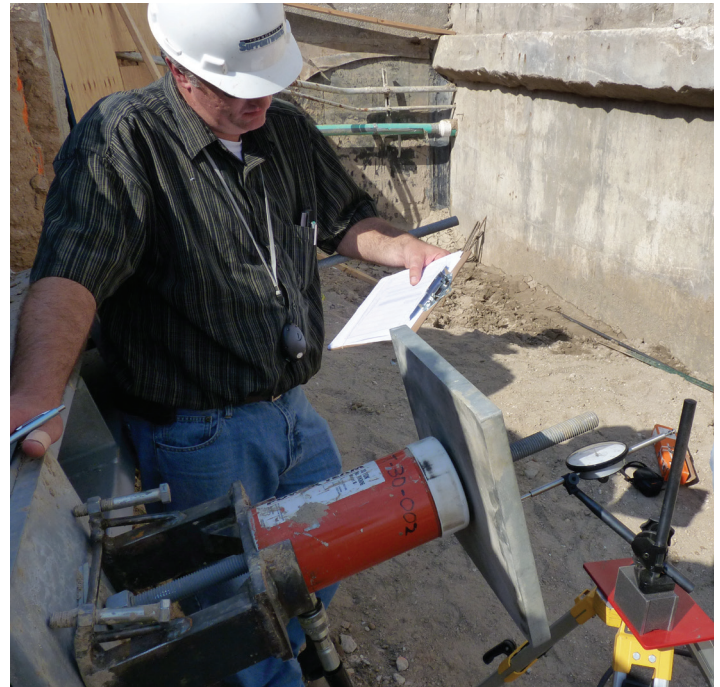
Pretensioning a Helical Tieback
