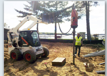
Advancing lead section of 3.5-inch O.D. pile
