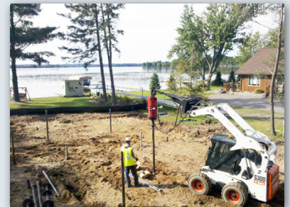
Piles advanced to refusal in the deep gravelly sand
