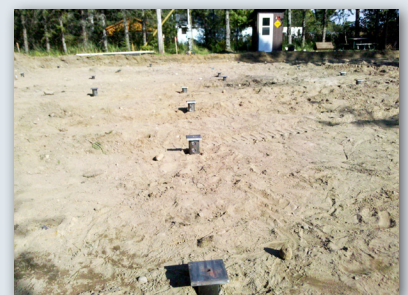
Completed piles and brackets
