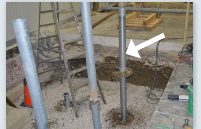
Advancing lead section
