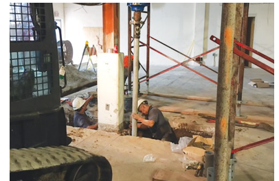
Connecting blank extension to lead section
