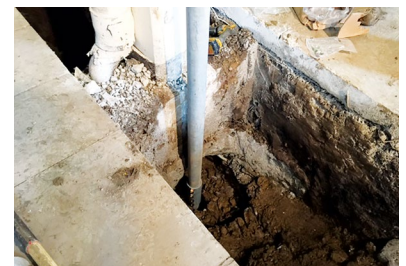
Pier advanced adjacent to column
