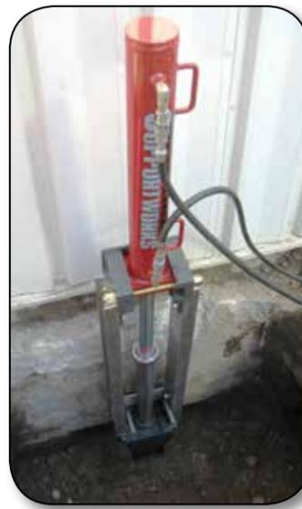
Hydraulic cylinder installing a 2-7/8 inch push pier.
