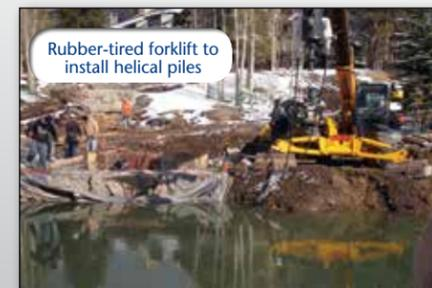
Rubber-tired forklift to install helical piles
