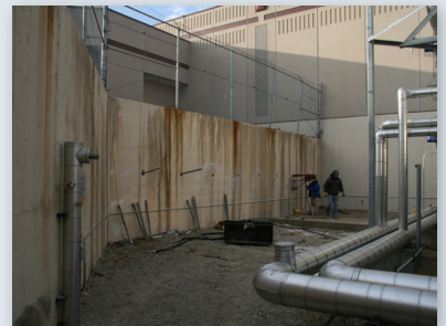
Tight access north side of wall; core-drilling 4" holes
