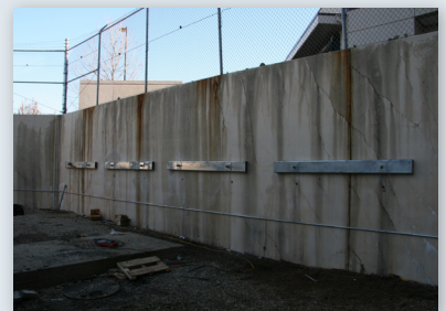
Tieback and water installation complete
