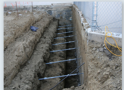
Tiebacks installed
