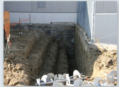
Soil excavated south side of wall
