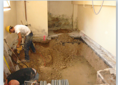
Limited access in area of proposed elevator pit
