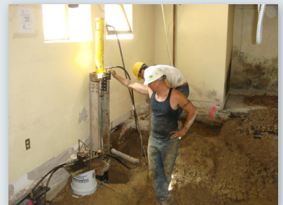
Piers driven to ultimate loads
