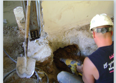
Footings notched and prepared for bracket installation
