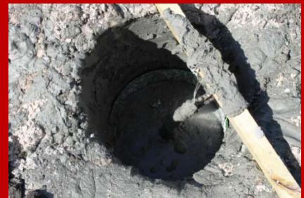
Each pile was 35-38 feet deep and 16 inches in diameter
