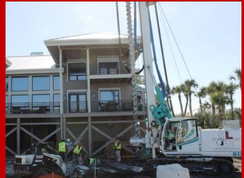
The 21 piles will provide support for an elevated pool structure being built
