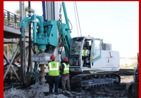
L.R.E. installed 21 Auger Cast piles
