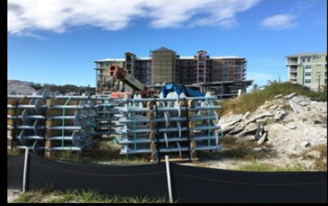
Galvanized Helical Piles waiting to be installed
