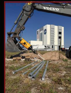
**NASA hired L.R.E. to install tie-back anchors**
