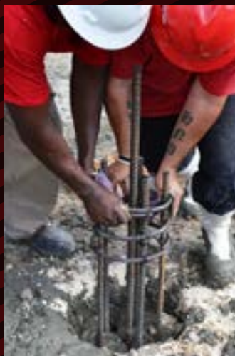
L.R.E. is a concrete expert and can manufacture its own steel cages.
