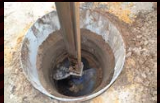
L.R.E.'s data acquisition system ensures the perfect pile every time.
