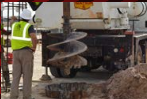
L.R.E. installs caisson and displacement piles.
