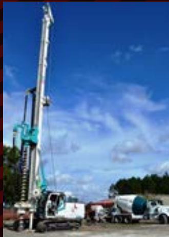
L.R.E. has specialized in large foundation projects since 1989.
