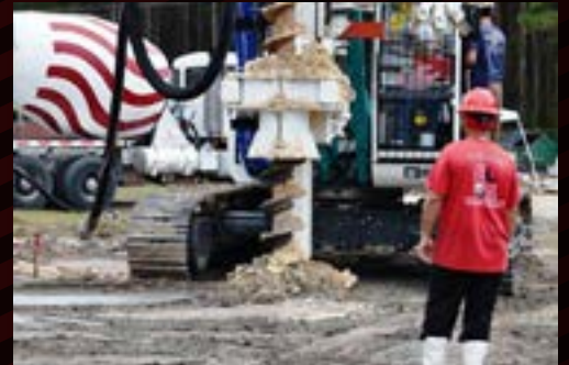
L.R.E. specializes in continuous flight auger cast piles.
