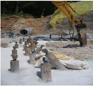
Micropiles are a small diameter replacement pile capable of supporting compression, tension, and lateral loading. The load capacity of a micropile is generated by the large cross-sectional area of reinforcing steel. Transfer of the load to the surrounding material is via the ground grout bond. This load transfer mechanism allows micropiles to be used in geologic conditions that would prove very diffi-
