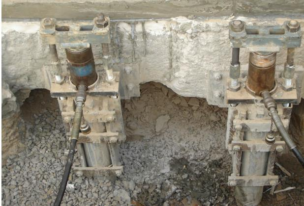
Foundation Specialties has been working with ECP for several years to develop an under footing bracket that can be used with small diameter micropiles. The ECP model 350 steel pier bracket can be installed and our MP250 drill feed used to install either hollow bar micropiles, or using a combination of continuous flight augers and down hole hammers a small diameter solid bar and cased micropile can be installed. The bracket allows for the structure loads to be directly transferred to the bracket.
